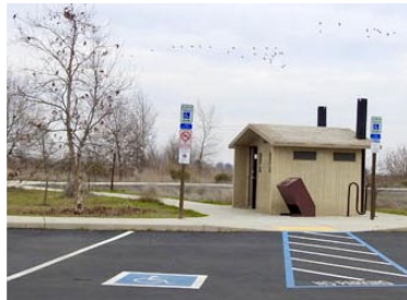
Accessible Restrooms at Stone Lakes
