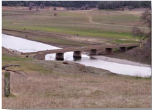
Salmon Falls Bridge
